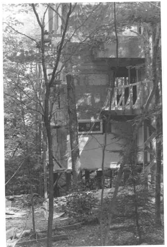
New construction on Fern Valley Road shows three adaptations to the steep slope; pilings minimize foundation excavations, a gangplank entrance eliminates cuts and fills, and a Clivus Multrum eliminates the possibility of septic contamination on the slope above the river.
