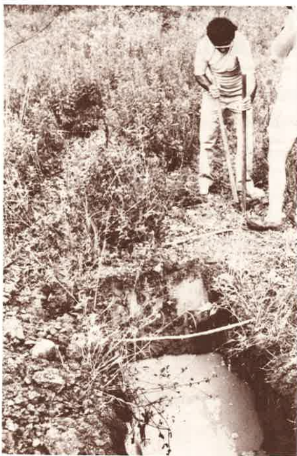
A standard percolation test is performed to predict the rate at which soil will absorb septic effluent.
