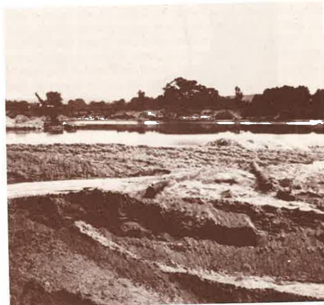
The gravel excavation at Broad Avenue and Weston Road reveals a picture of a typical stratified drift aquifer deposit.
