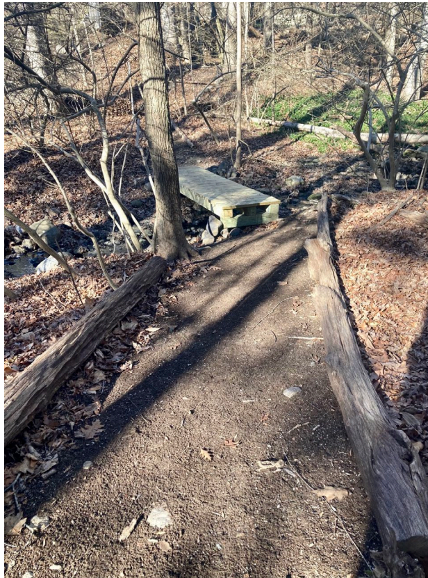
Northern Trail Bridge
