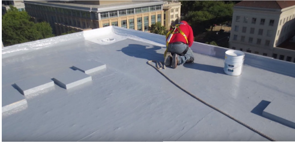
Photo by Reliable Roofing
