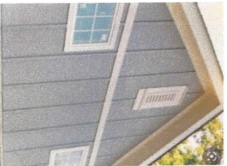
Board 4' & Batten-1 1/2' Hardie Cement Board
