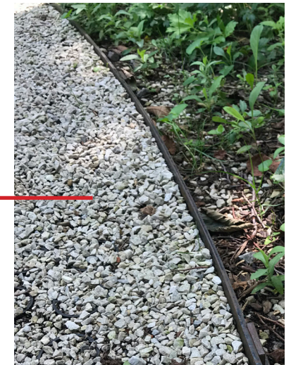
Porous paving & metal edging
