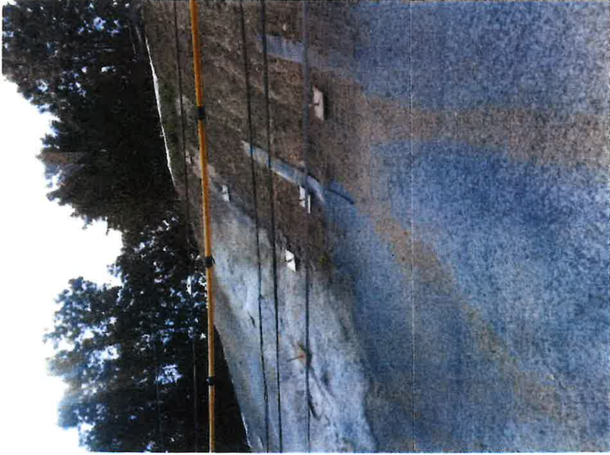
Typical Soil Nail Construction
