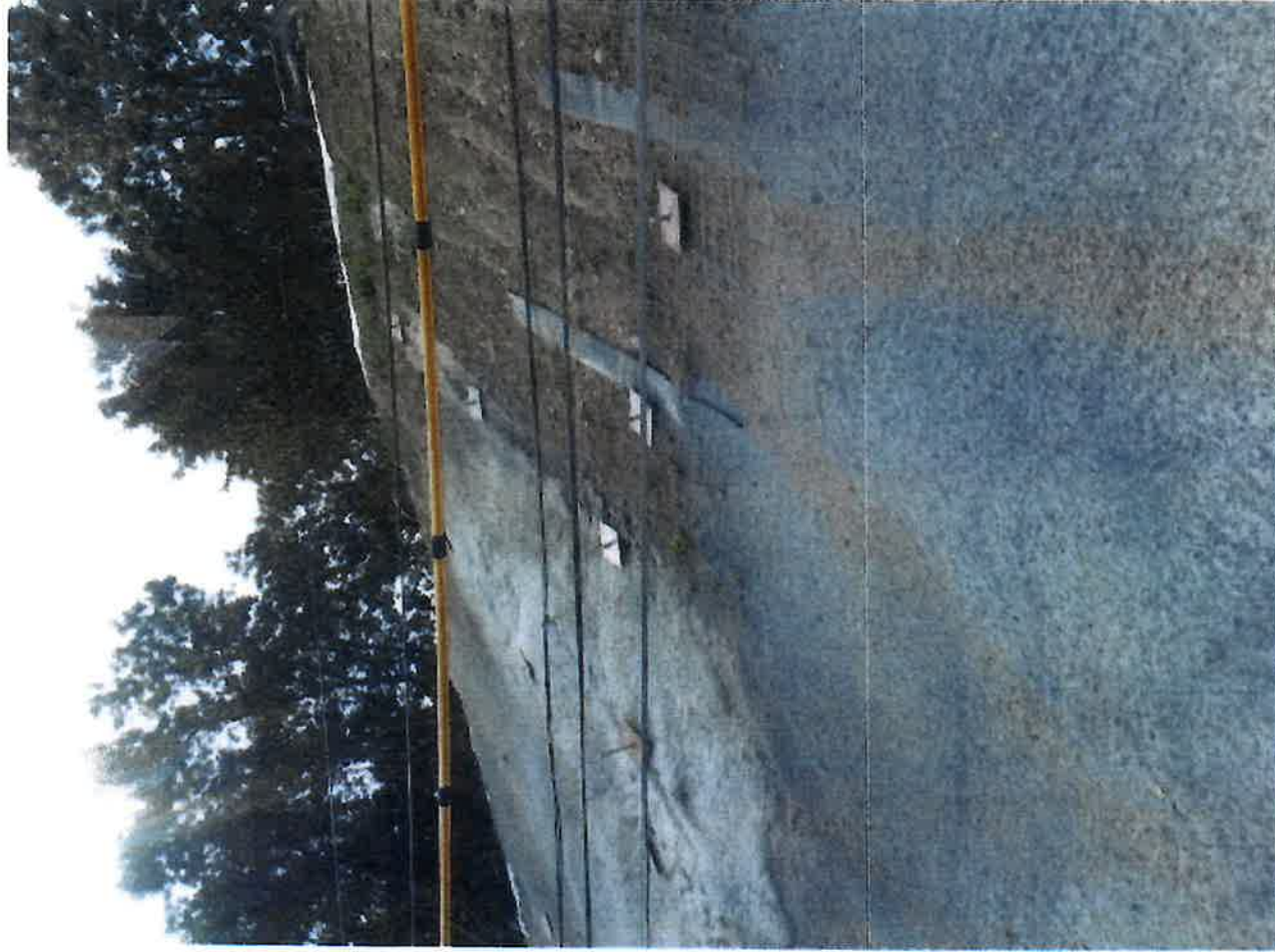
Typical Soil Nail Construction
