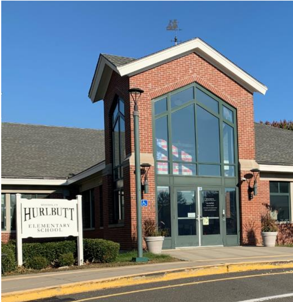
Hurlbutt Elementary ~ 24 School Road
