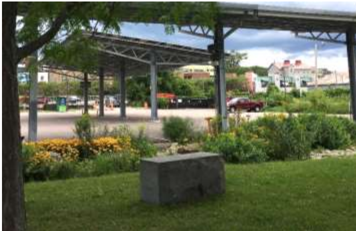
Solar panels and bioswale for parking lot
