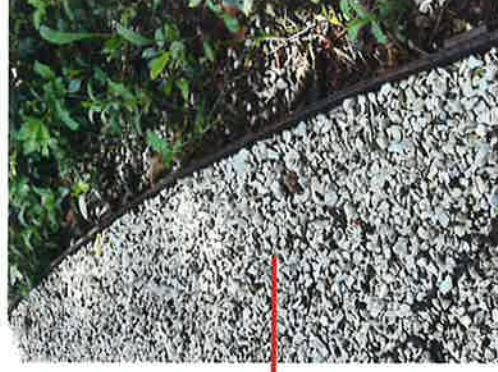
Porous paving & metal edging
