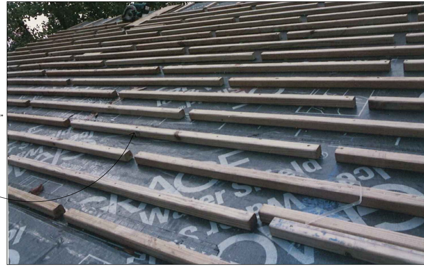
B SHINGLE LATH SPACING R3 (2010 PROJECT)
