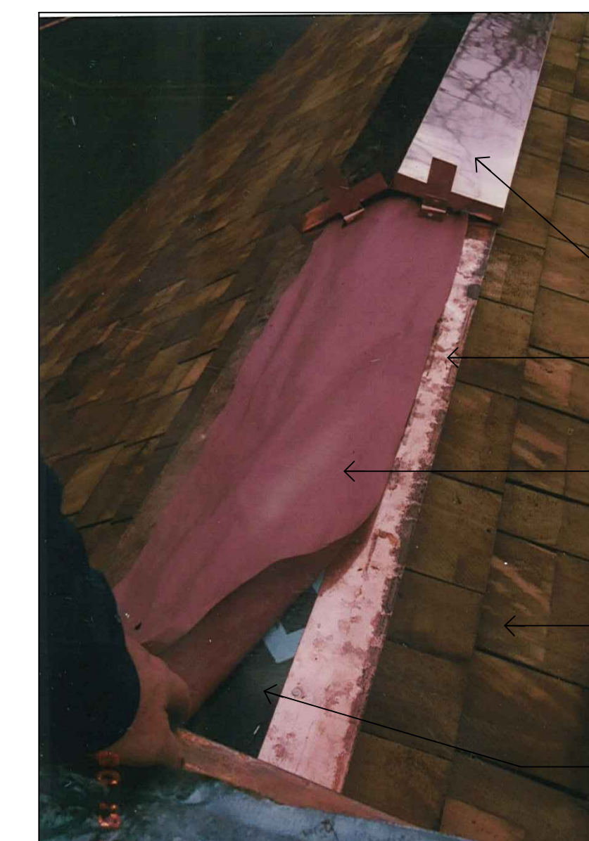
H RIDGE CAP INSTALLATION R3 (2010 PROJECT)
