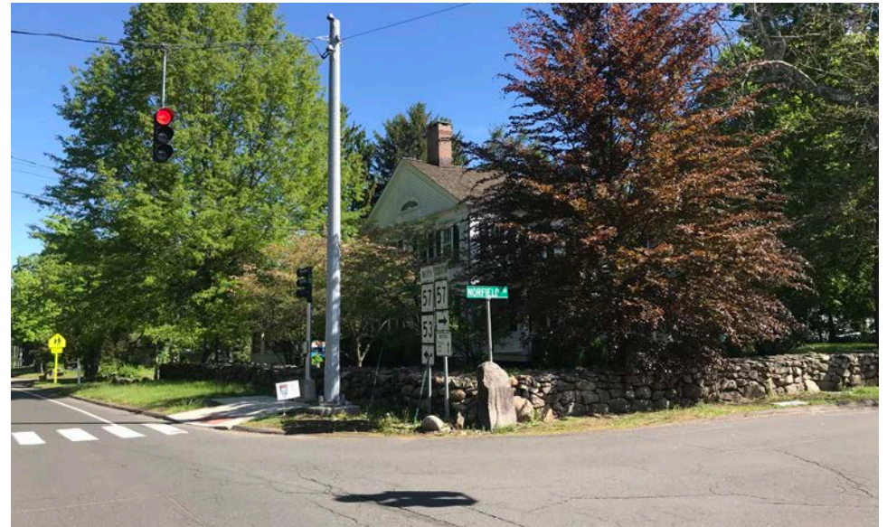
Accessible Drop Ramp without Sidewalk Connection at the Corner of RT 57 and Norfield Road
