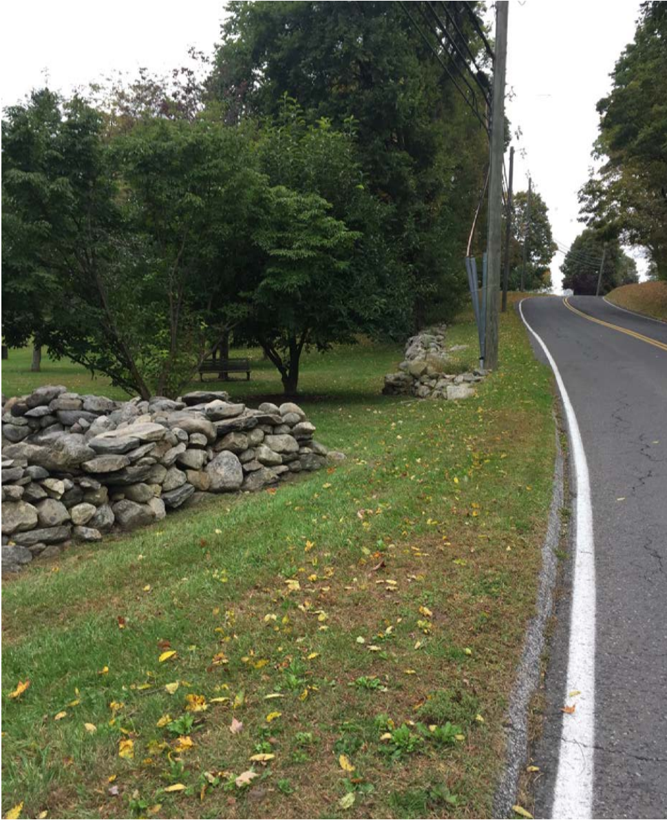
Horizontal & Vertical Road Alignments and a Lack of Roadway Shoulder Limit Safe Bicycle Activity
