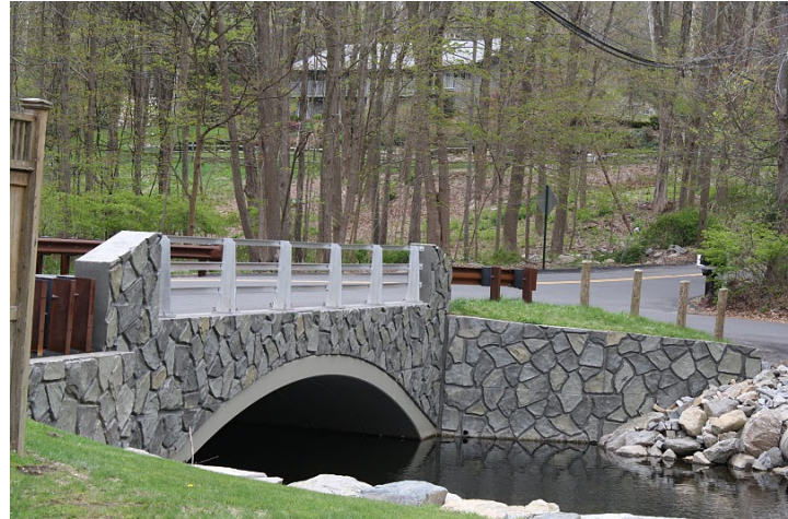
Cartridge Road Bridge
