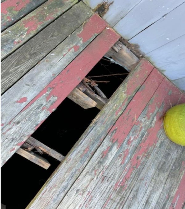
Northern deck in need of repair
