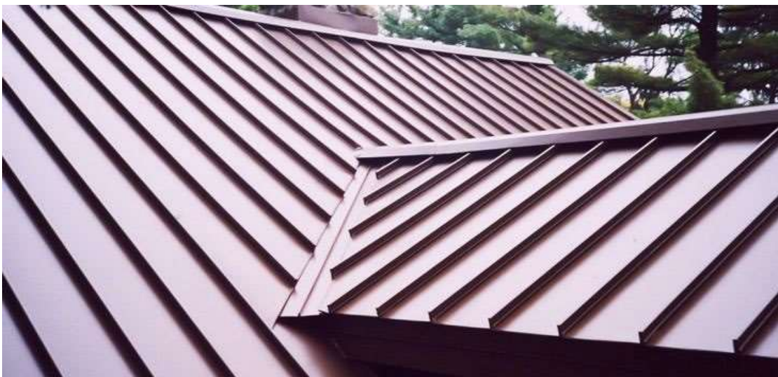
Photo by Classic Metal Roofing Systems
