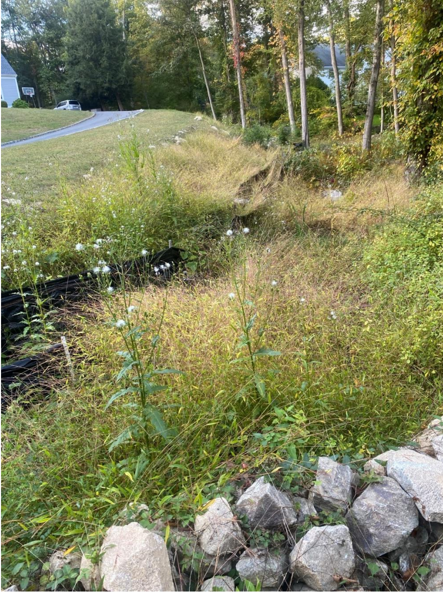
Filled area left, silt fence, wetlands right looking north
