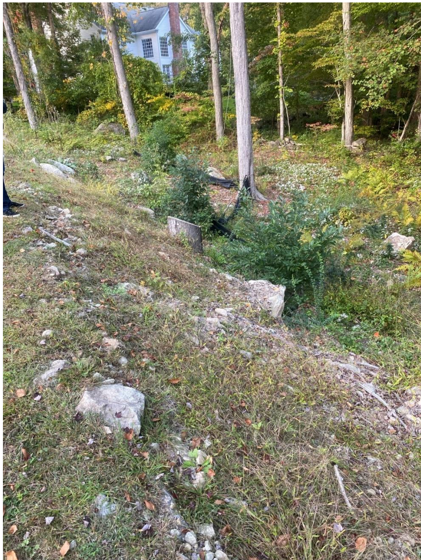
Further up filled area slope steepens to approximately 1 to 1.
