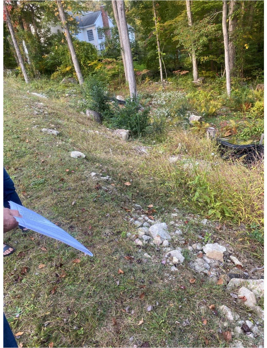
Slope to silt fence approximately 1 to 2 lower area near wetlands
