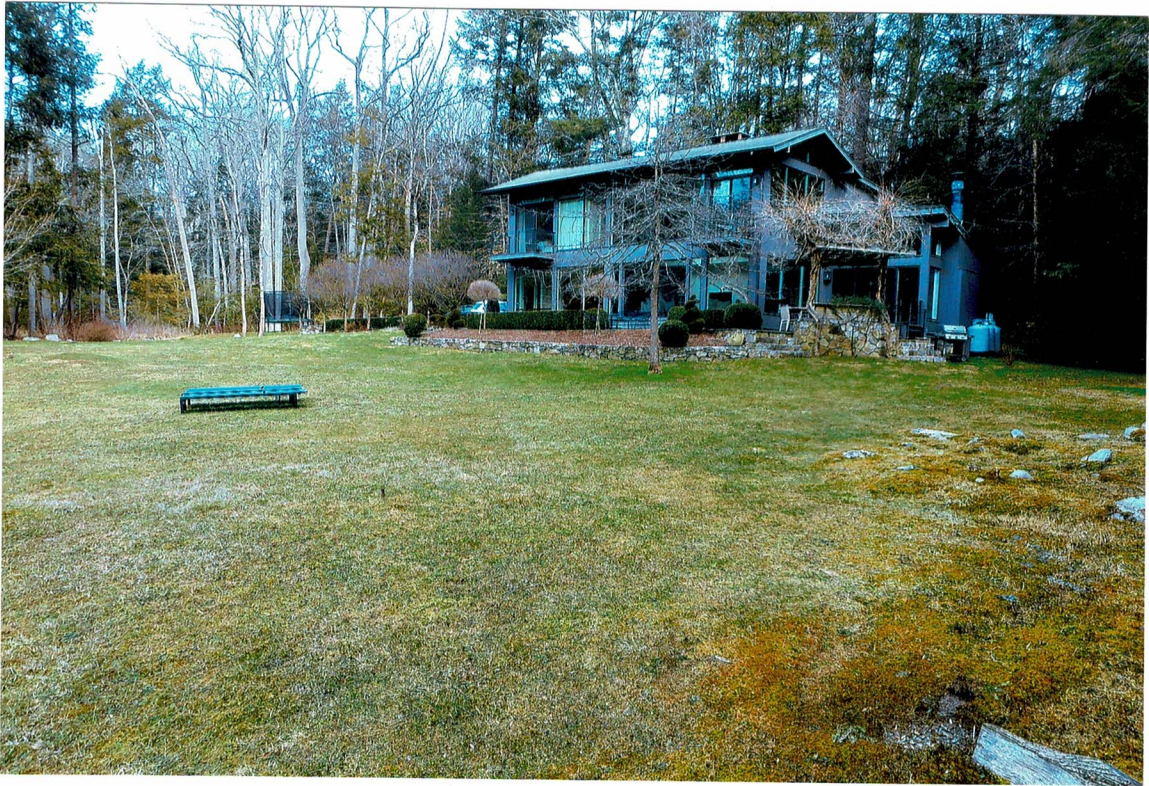
Photo 4 Looking northeast and upslope across lawn and toward residence.
