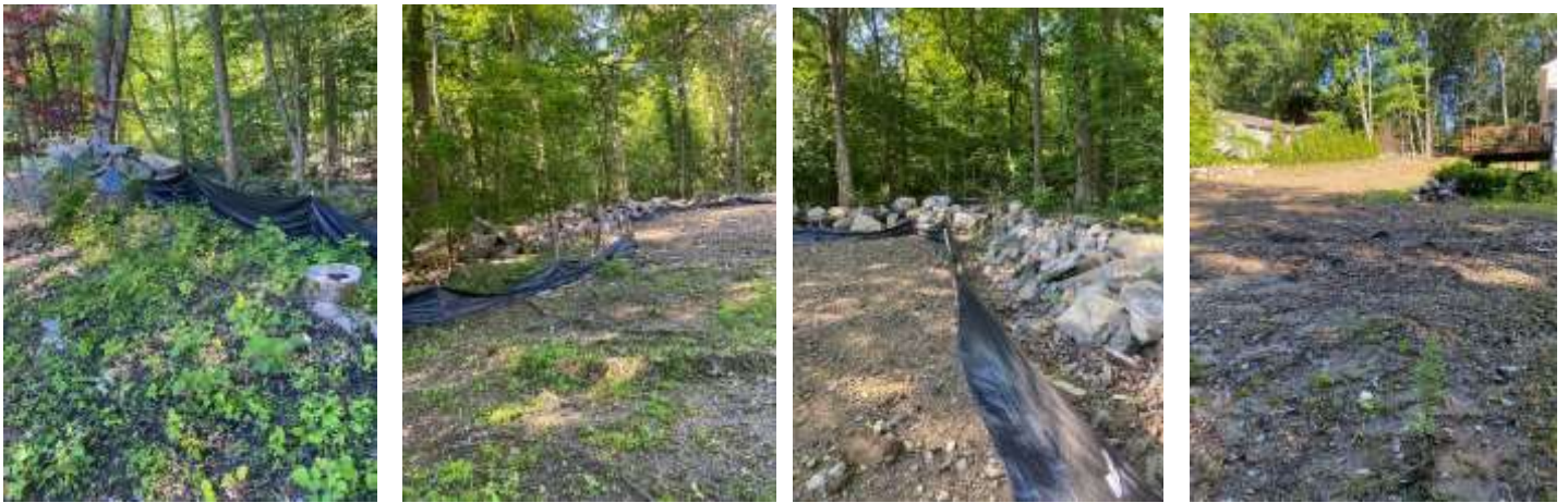
Cleared areas photos 8 Jana - 1, 2, 3 and 4
