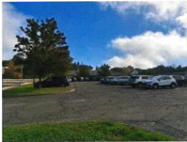
7. View of School Parking Lot.jpg
