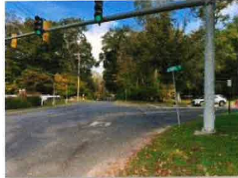
2. View Looking North.jpg
