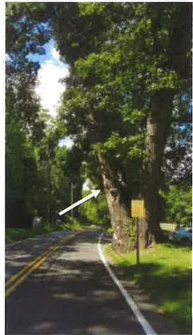
Leader immediately adjacent to road, damaged by vehicle impacts
